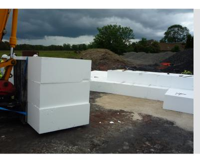
Filcor (Expanded Polystyrene) is increasingly being specified for an ever-growing range of applications. The most common applications include use as a lightweight structural fill alternative to more traditional fill materials or as a lightweight void former in structural concrete.
