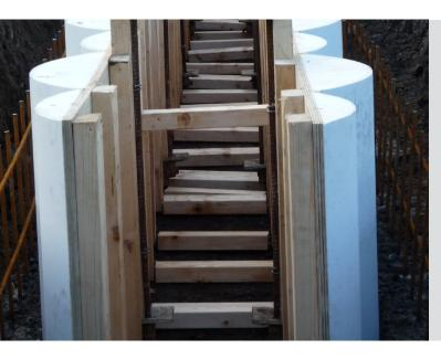
Cordek Reusable Guide Wall Formwork is used to accurately form an insitu concrete guide wall which is critical in the positioning and alignment of piles in a contiguous and secant piled walls.
