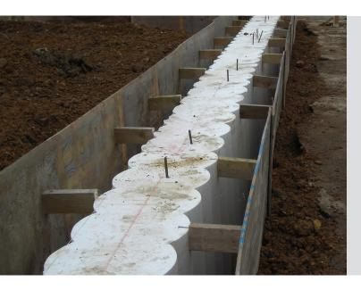
Sacrificial Guide Wall Formers are used to accurately form an insitu concrete guide wall which is critical in the positioning and alignment of piles in a contiguous or secant piled wall.
