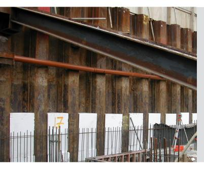
Sheet Pile Infills are designed as a quick, economical and lightweight solution to infilling the open pans in an exposed sheet pile wall.
