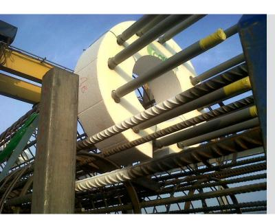
Corbreak is a unique system to aid the trimming down of piles. During the construction of piled foundations, it is quite often necessary to reduce the height of the piles and expose the reinforcement within them. The removal of concrete required to do this has been traditionally carried out using hand held tools which subject the users to a number of health and safety related issues e.g. noise and vibration.
