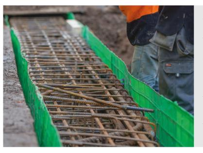
The Cordek Corgrid system is designed to provide an economical permanent formwork system for the construction of reinforced concrete ground beams, pile caps and other associated cast in-situ structures.
