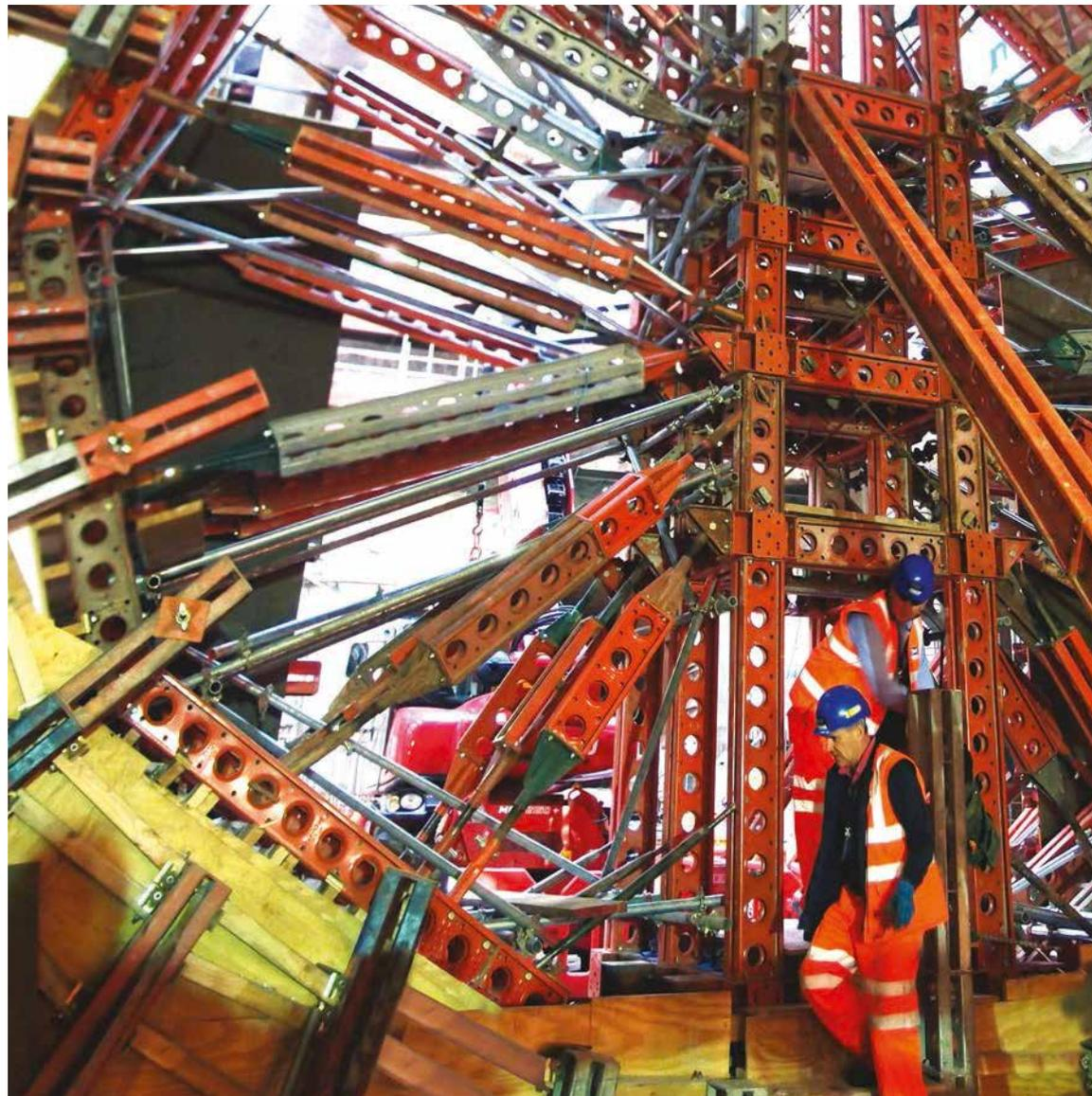
steel Slimshor frame, providing support to the outer formwork. Cordek then created a 3D CAD model of the angled tunnel intersection and designed the profile of the formwork required.
