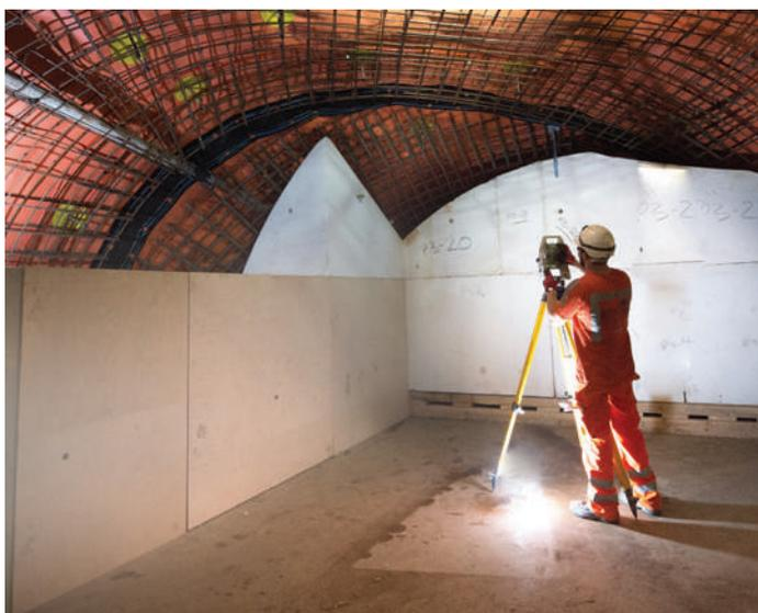
**The formwork concept was installed in stages to suit the preferred concrete pour sequence required for this complex structure**
